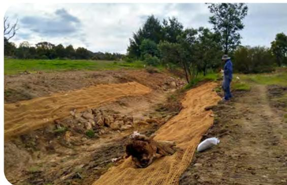
**After** – Banks battered and covered with coir mesh to facilitate plant growth and protect soil from further erosion. Instream rock structure (left) and rock ramp (top) work to slow water flow.
