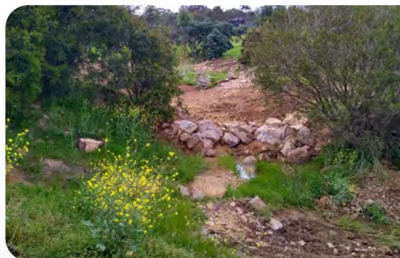
**Rock ramp** – Designed and installed to slow water flow before it enters the pond below.
