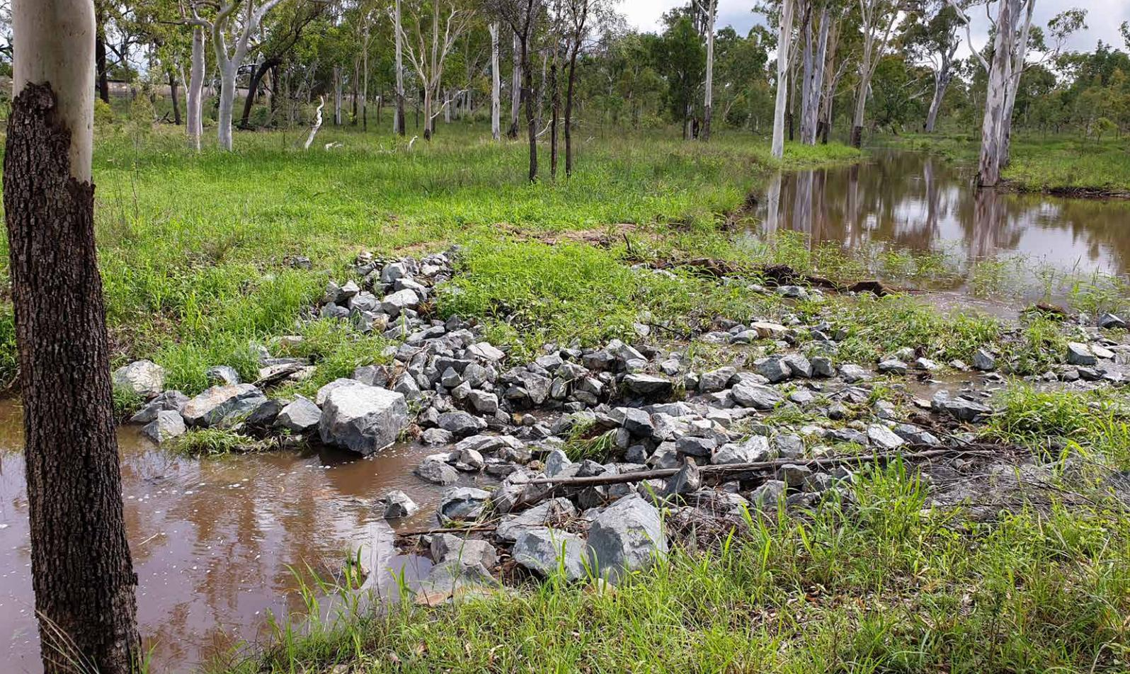
TOP: Leaky weir being constructed at Mt Pleasant Learning Hub, September 2019. BOTTOM: Leaky weir after rains, February 2020.
