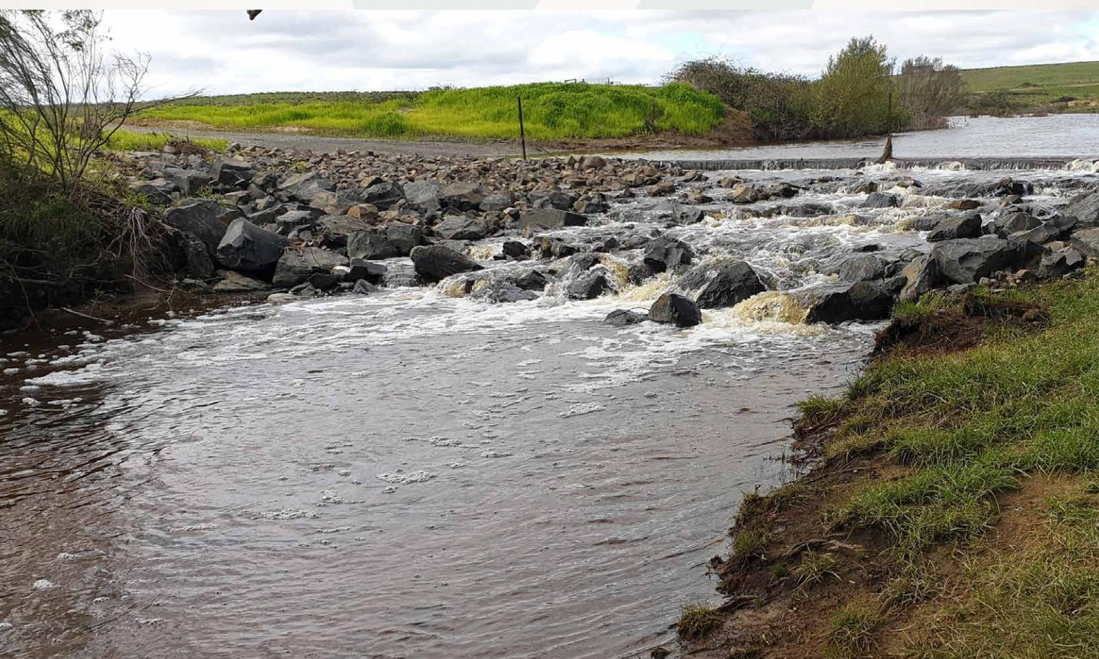
TOP: Leaky weir being constructed at Duralla, February 2020. BOTTOM: Leaky weir after rains, March 2020.
