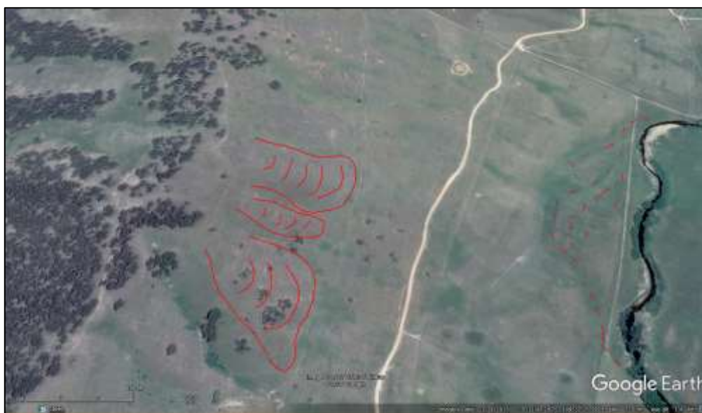
Figure 22. Soil environments driven by geomorphic processes. Ridgeline / crest along tree line (LHS); colluvial deposits (fans) downslope and meandering paleo-channels clearly visible in the floodplain
