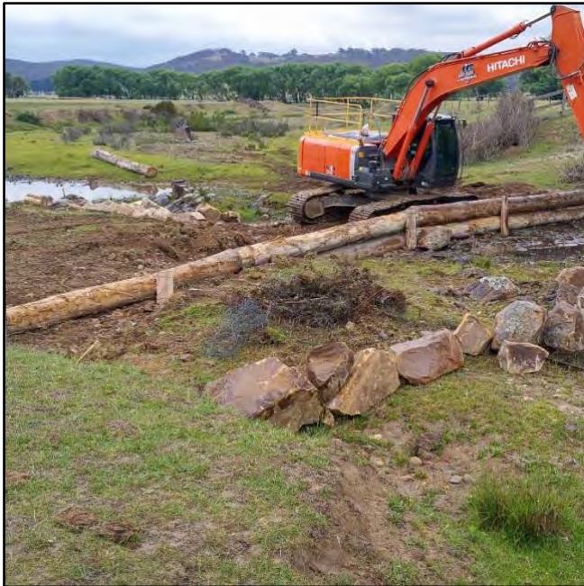
Figure 38: Implementing in-stream structure late 2018
