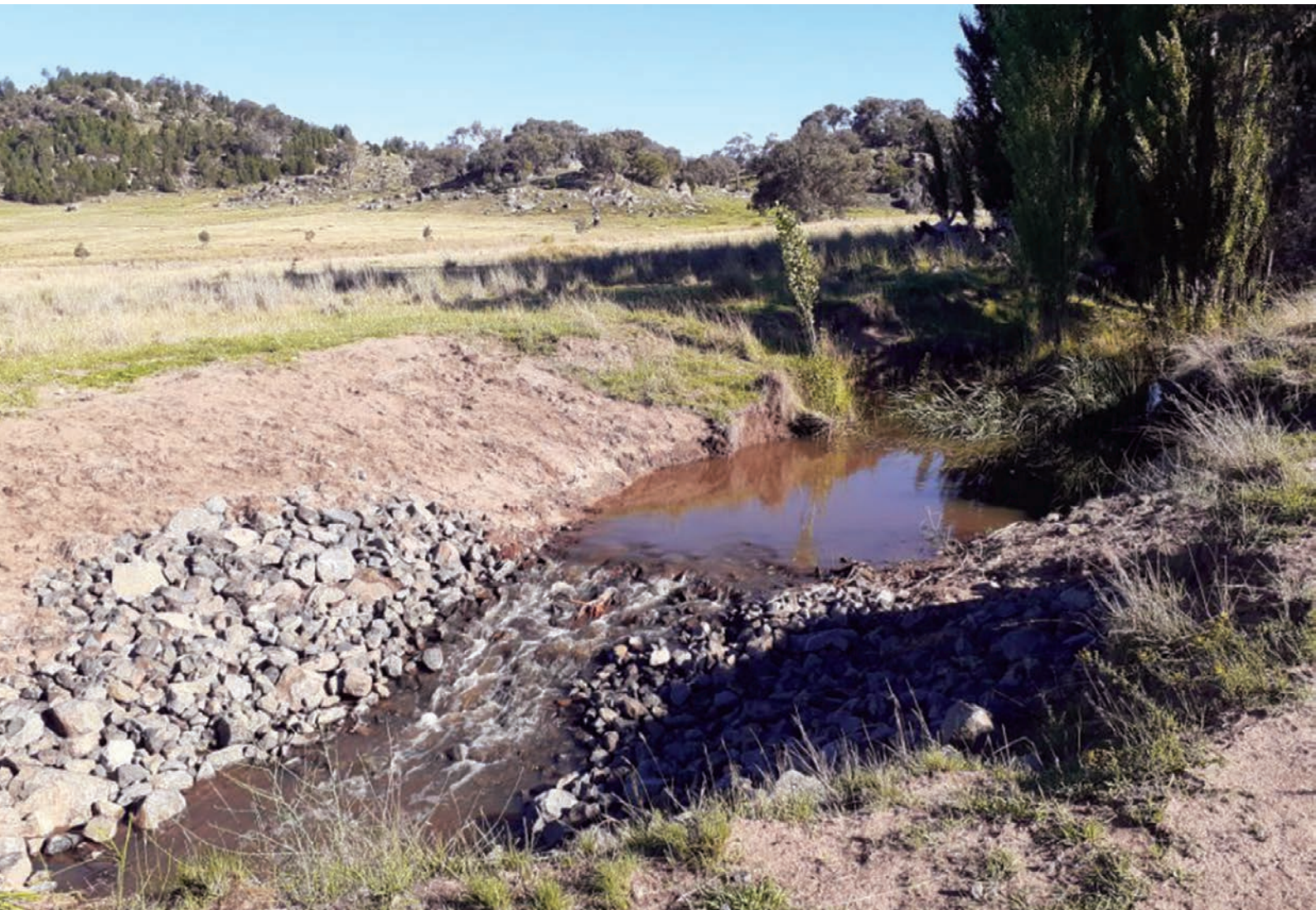
Above: Construction of a rock chute at Cadfor
