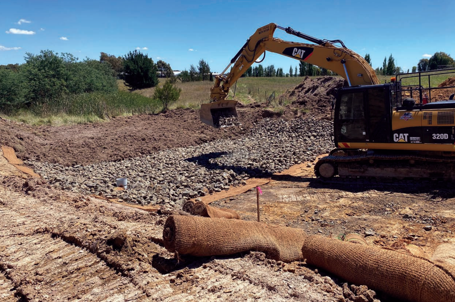
Above: Construction of a rock chute at Cadfor
