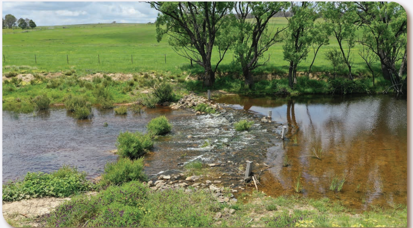
Figure 67: A log-sill and rock weir.
