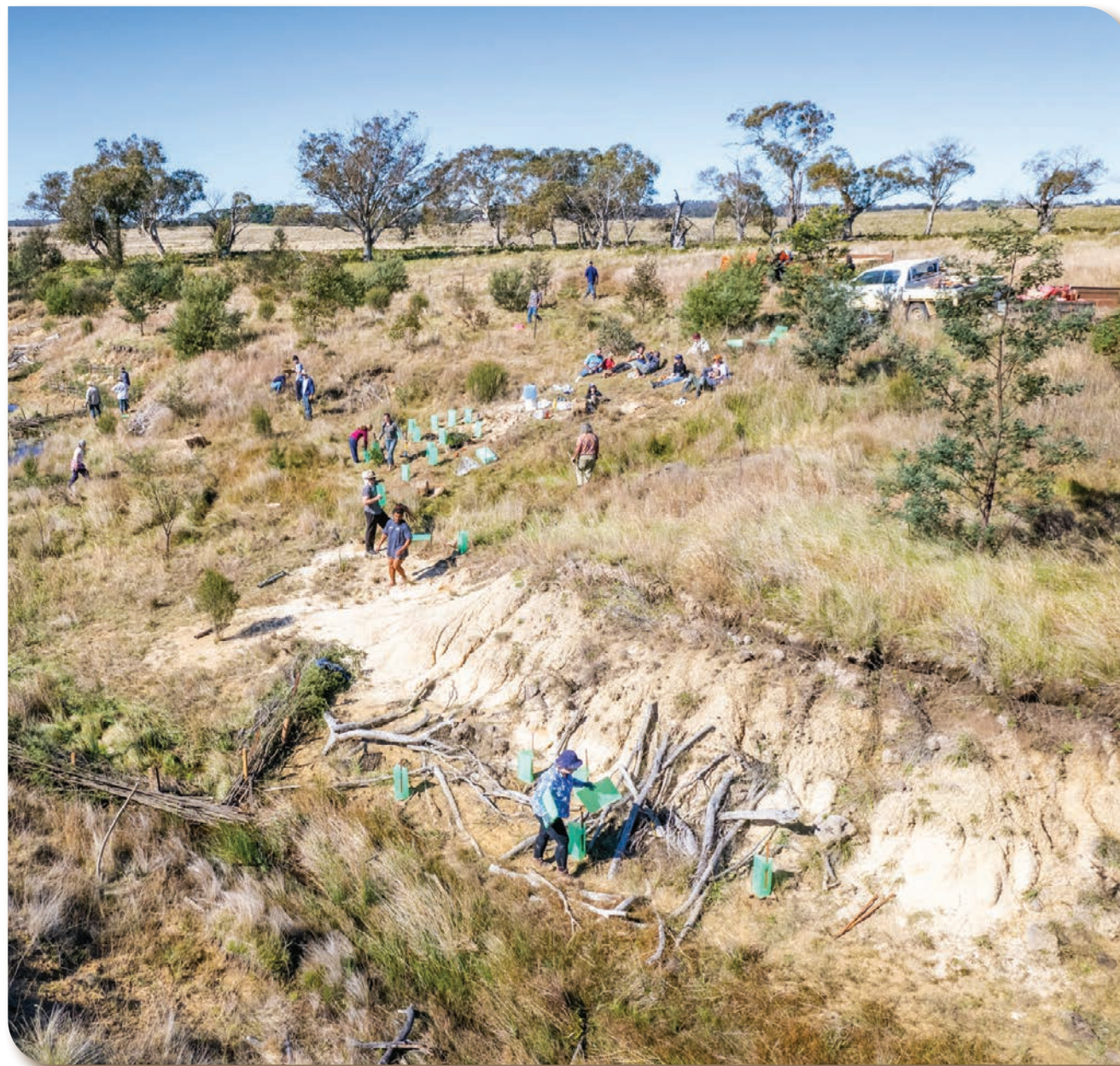
Figure 55: Brushpacks being installed in a large erosion gully. Photo by Grow Love Project
