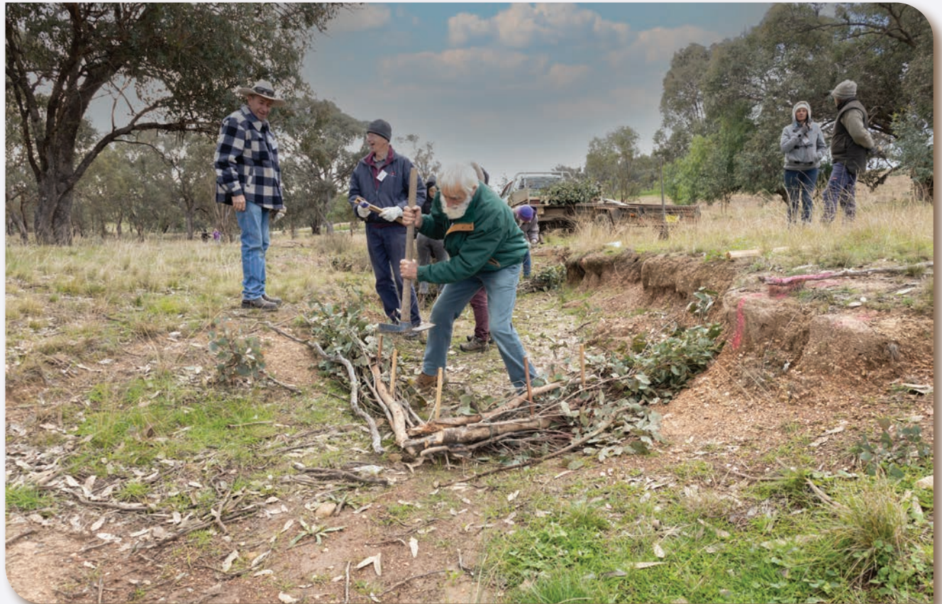
Figure 63: A brushpack being installed in an erosion gully.
