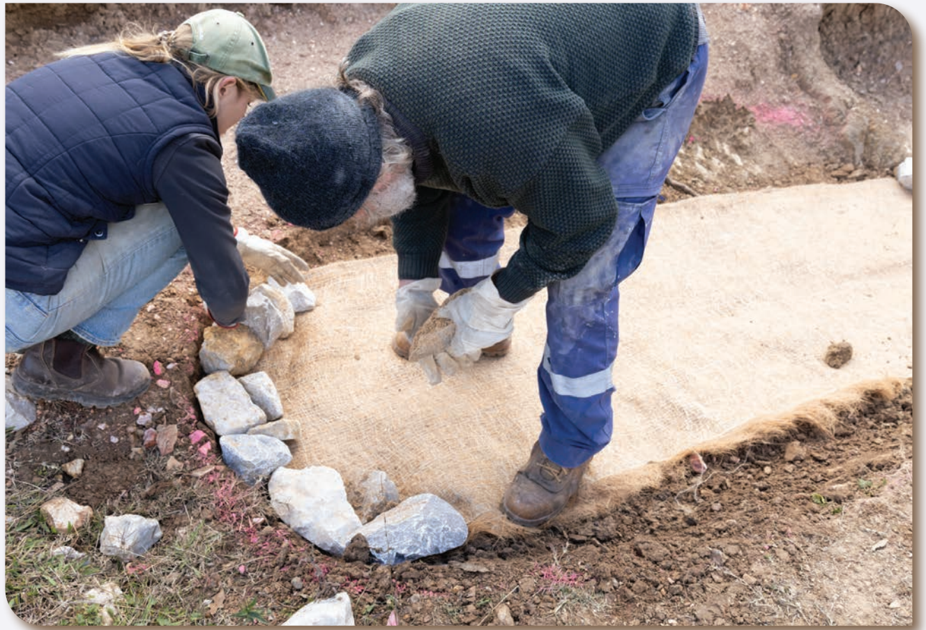
Figures 66a and b: Rock armouring structures being installed in erosion gully. Photo by Maddison O'Brien.
