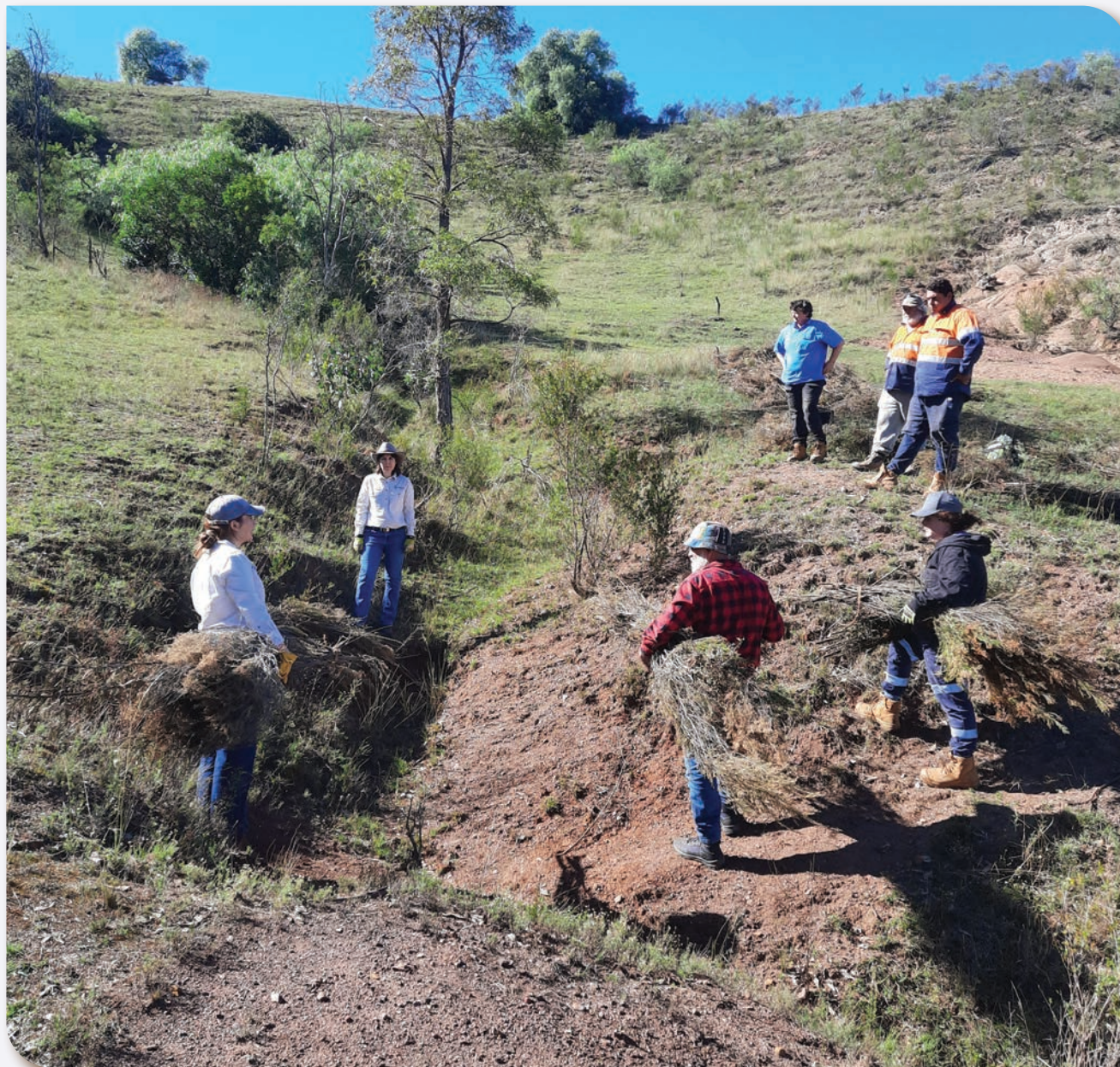
Figure 54: A North East Wiradjuri Company team prepare to install brushpacks in an erosion gully.
