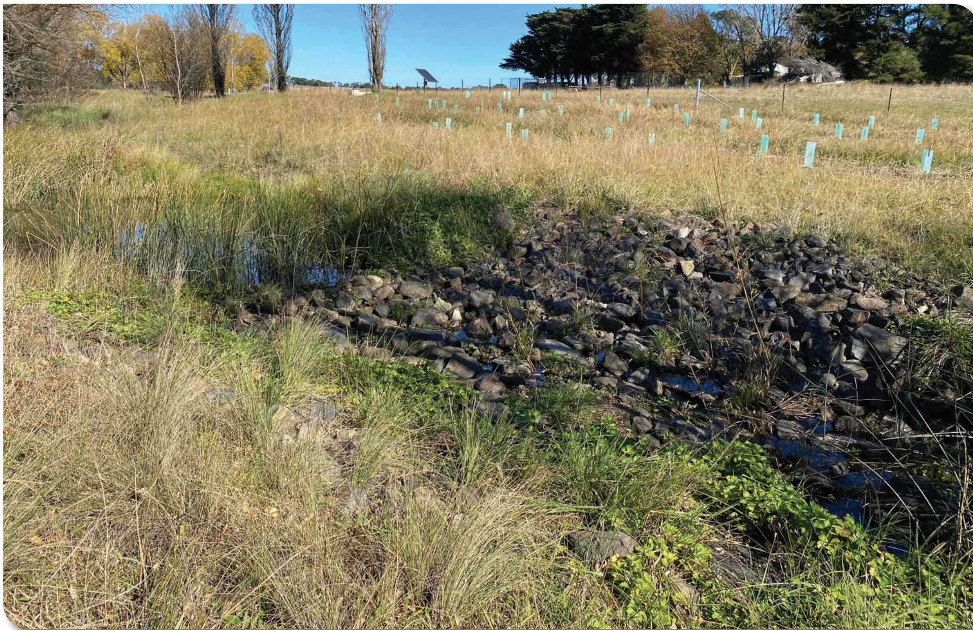
Figure 53: A waterway with a recently completed rock weir, behind which a new pond has formed. New riparian fencing to exclude stock, and new plantings are contributing to the regeneration of the site. Emerging plant communities are visible on the structure, banks and in the pond. See Lorrina case study, page 110.
