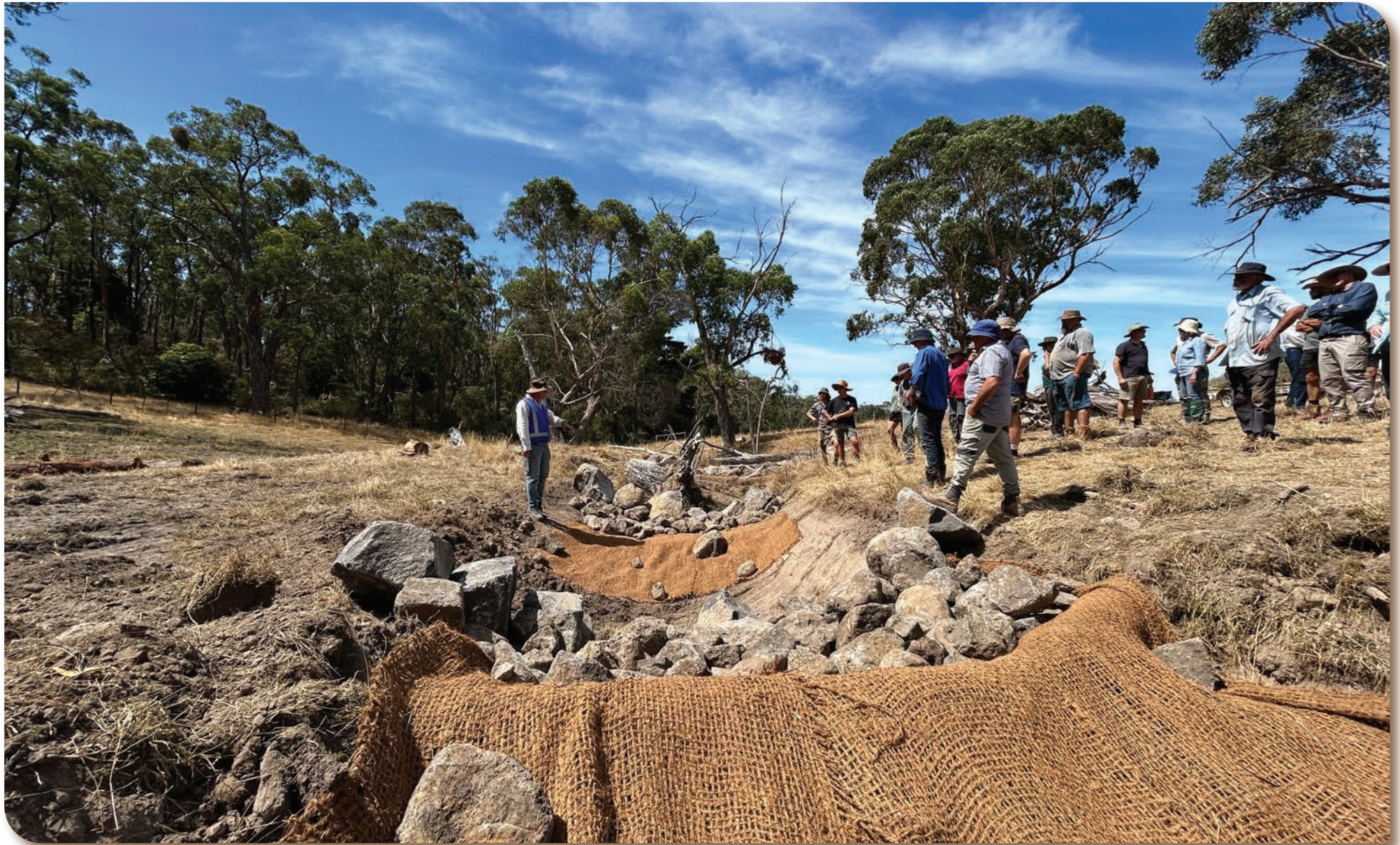
Figure 51: A series of rock weirs being installed in an erosion gully at a landscape rehydration skills event.
