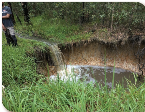
Figure 84: An active headcut in one of the drainage channels
