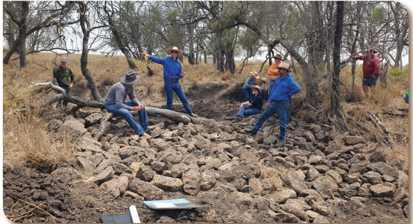
Figure 40: An erosion gully in which a rock weir has just been installed. The weir will slow flood flows, prevent further erosion and start to rebuild the gully floor by causing ponding and deposition.
