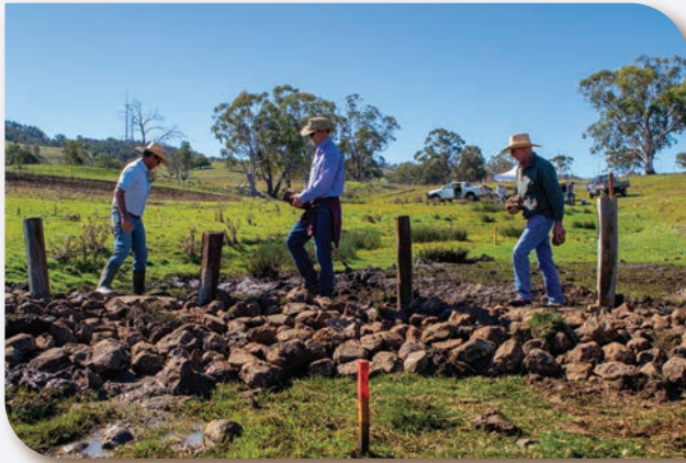
Figure 93: Log-sill and rock weir being constructed during the bootcamp. Photo by Grow Love Project.
