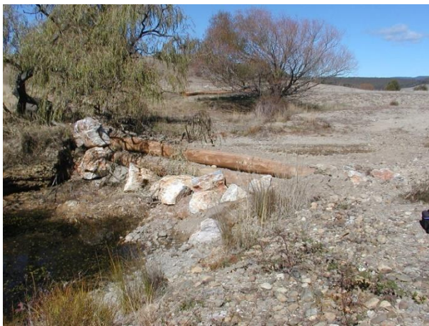
Figure B4: Example of a log sill with large rock anchors.
